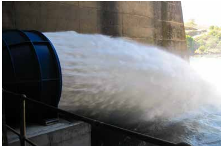
DN 1400 fixed cone discharge valve with hood
