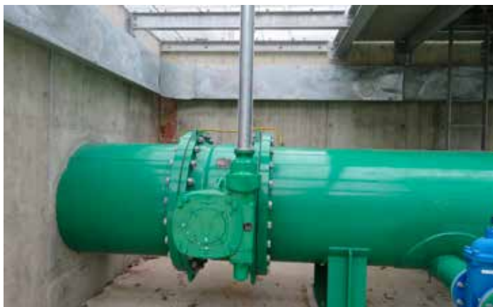
DN 1400 fixed cone discharge valve with hood
