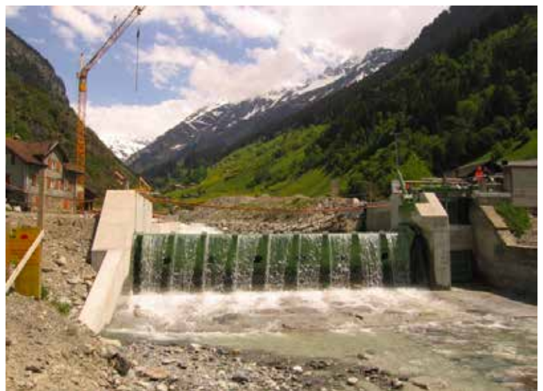
CREST GATE 16 mts wide - Backed up water level 2.5 mts
