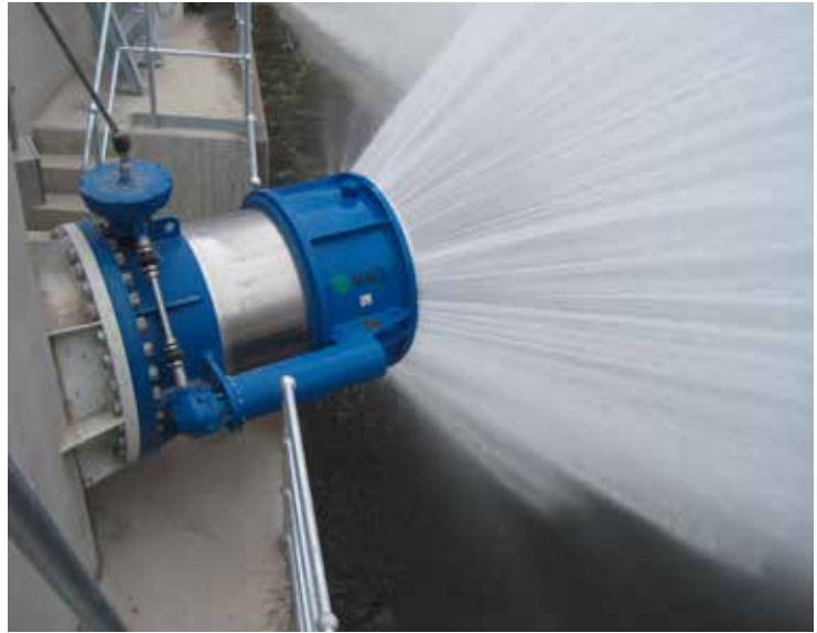
DN 900 PN 25 Fixed cone discharge valve at a dam in Canberra Fixed Cone discharge valve the KSS plus manufactured size range from DN 400 to DN 2000
